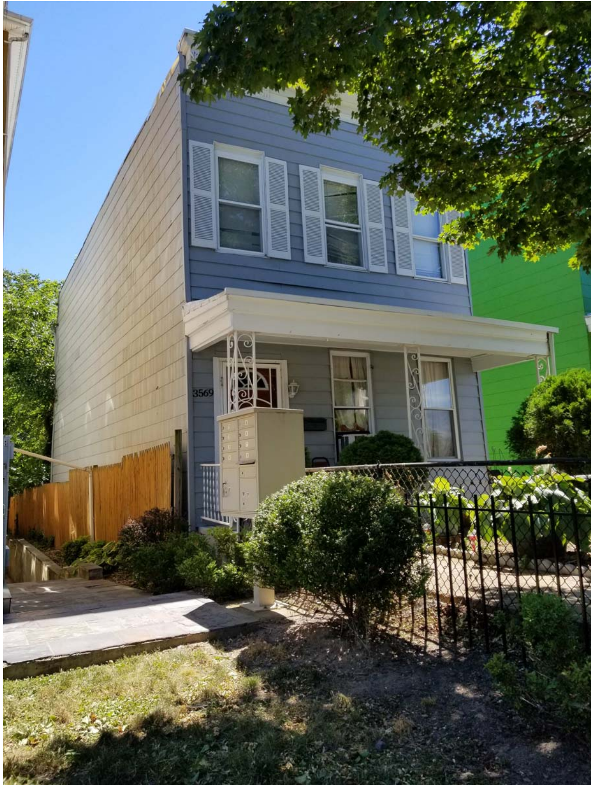
EXISTING FRONT PORCH CONDITION
